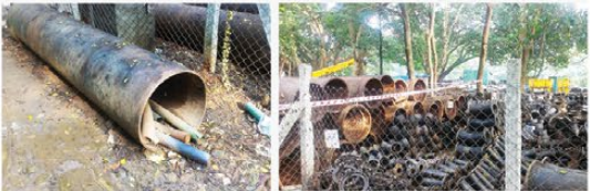
To the left is an image of cast iron pipes which have been partly corroded, abandoned beside the BWSSB building at Krishna Rao park to be picked up by dealers of scrap metal. This design proposes treating the pipes for corrosion removal and treatment and powder coating the pipes red for reuse.
